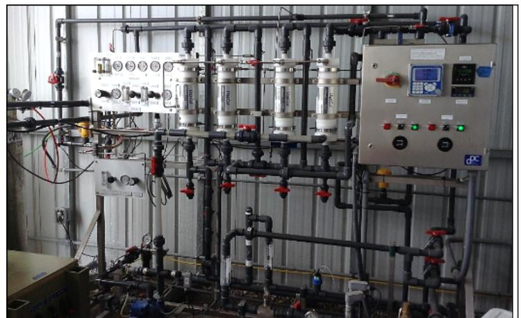
Figure 10. Four Membrane Contactors in Series to Provide up to 4-Log (99.99 Percent) Removal of Dissolved Oxygen (courtesy of City of Clearwater, 2014)
